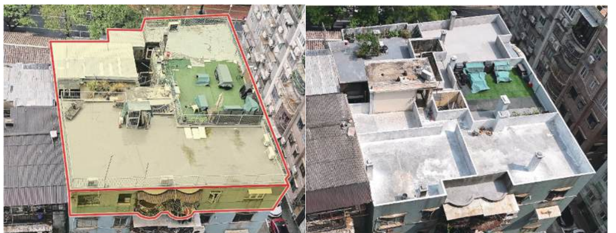
This undated handout combination of two photos provided yesterday by the Land and Urban Construction Bureau (DSSCU) shows the site before (left photo) and after the removal of its illegal brick wall and metal-roofed rooftop structures.
