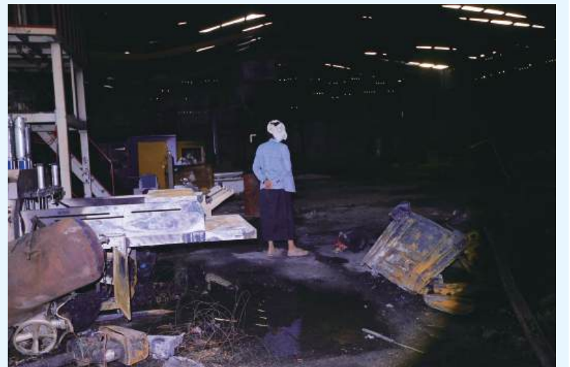
A Yemeni man inspects melted foam inside a factory after a strike that Houthi authorities-run media attributed to Saudi Arabia, in the Shamlan neighbourhood of Yemen's capital Sanaa yesterday.
