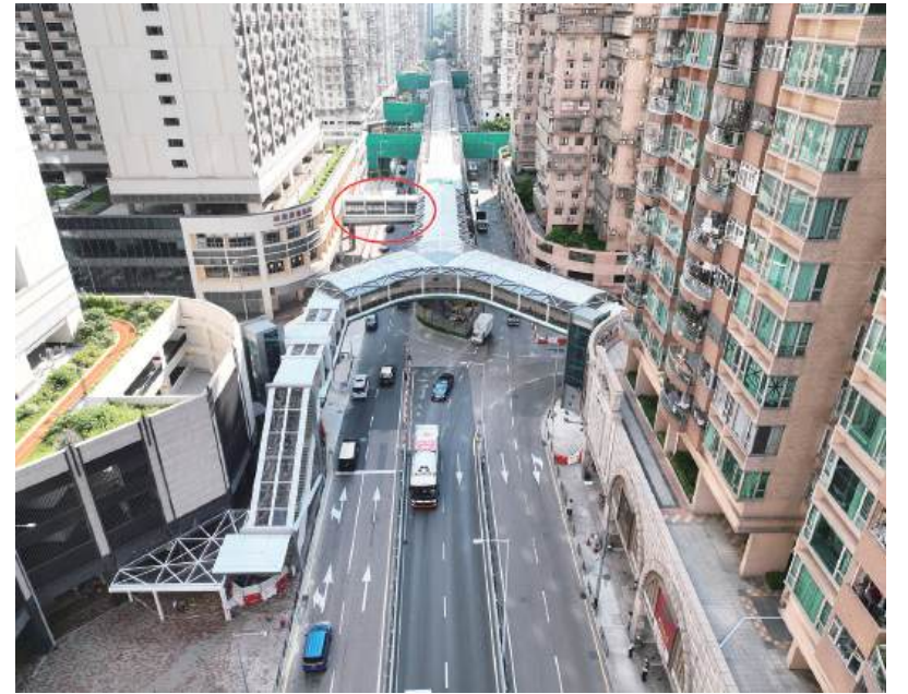
This DSOP handout photo released on Saturday shows the ongoing skywalk project on Avenida do Nordeste. Two access points (bottom) and the footbridge (red circle) connecting to the seniors' rental housing estate will open today.
