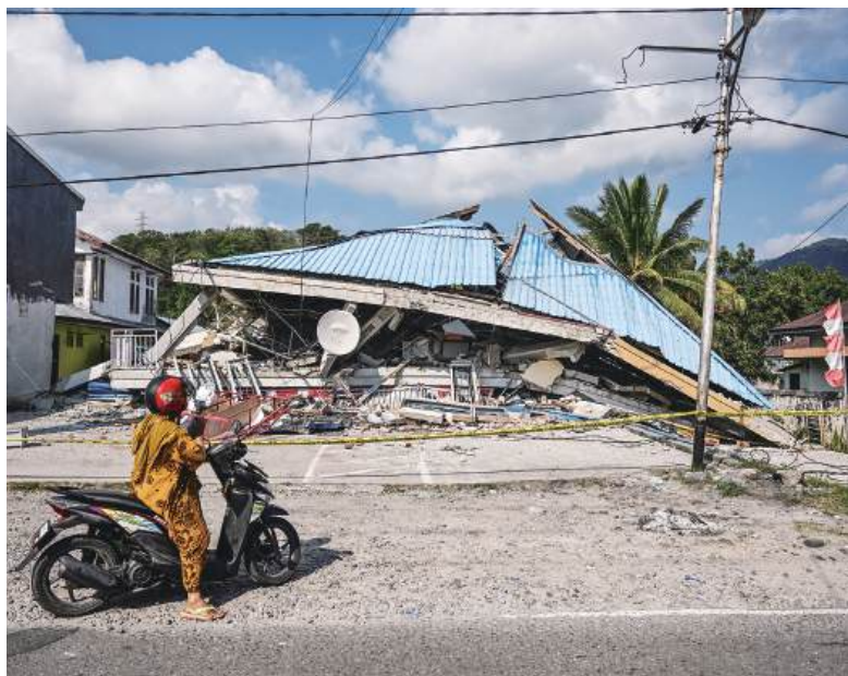
A motorbike stops next to a collapsed building following a 7.7-magnitude earthquake in Borong, East Manggarai, East Nusa Tenggara yesterday. Help started arriving yesterday for thousands of evacuees on Indonesia's Flores island after a powerful earthquake killed 53 people, injured dozens and damaged hundreds of houses and buildings. – AFP
