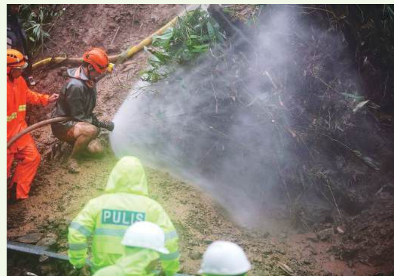
Rescuers use a water-hose to clear mud amidst rubble as they search for survivors after a rain-drenched mountainside collapsed on several houses in Baguio City, north of Manila yesterday. – AFP
