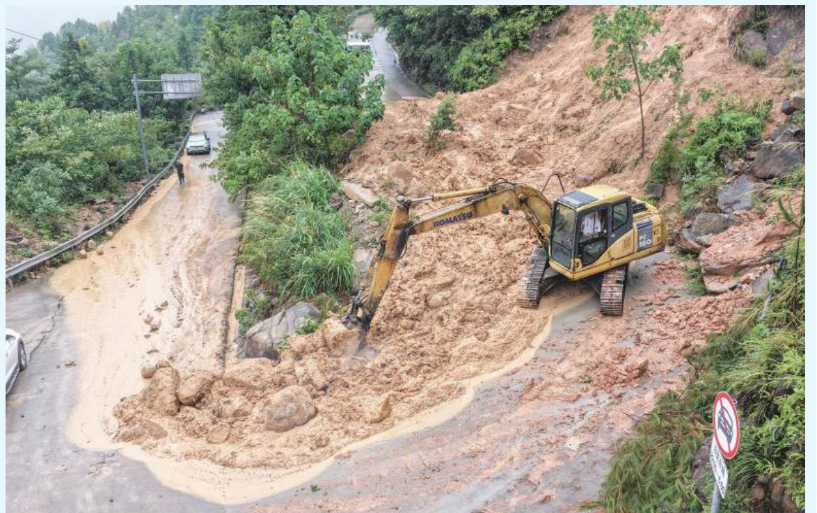
A drone photo taken yesterday shows a staff member operating an excavator to clear a collapsed section of a road in Luojialiao Village in Wenzhou, Zhejiang Province. Typhoon Dolphin is moving inland after making two landfalls along the coast and is expected to bring heavy precipitation to more than 10 provincial-level regions, according to the National Meteorological Center yesterday.
