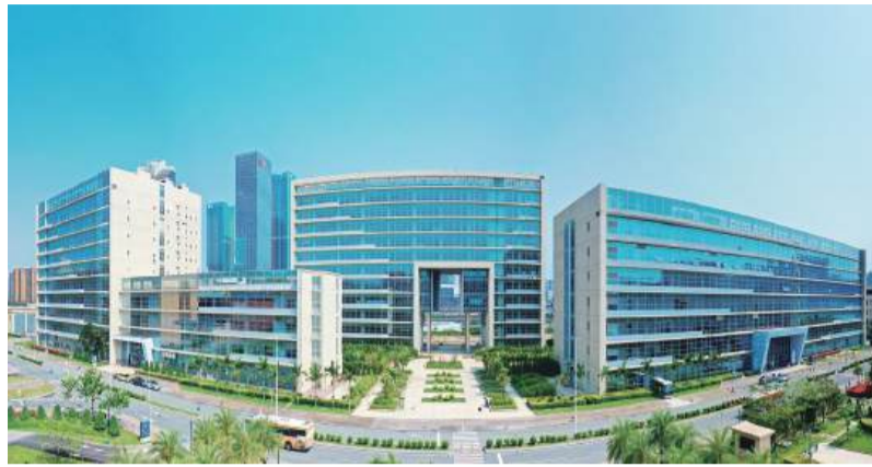
This undated handout photo provided by the public University of Macau (UM) recently shows its scientific research base on its campus in Hengqin.
