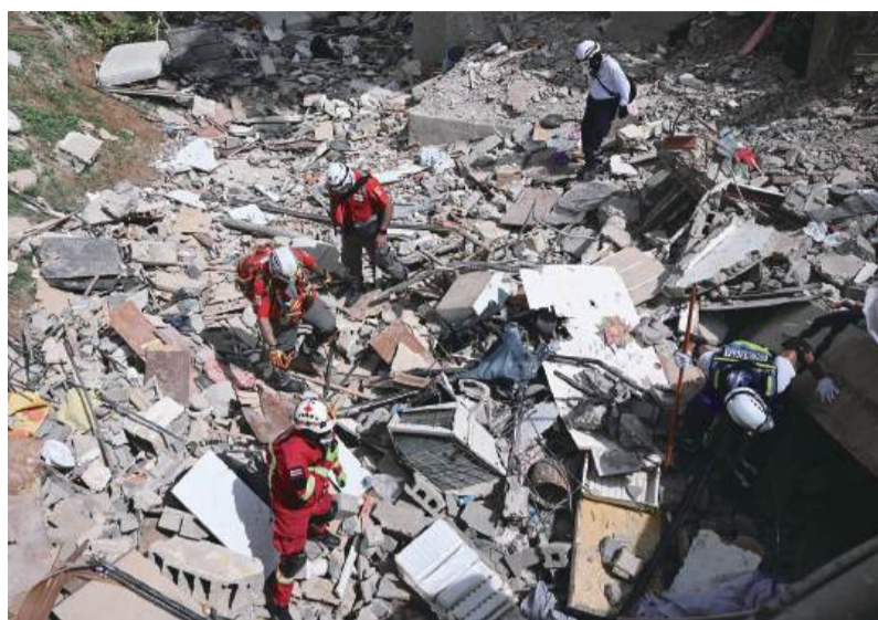
Costa Rican rescuers search through the rubble of a collapsed building in Catia La Mar, La Guaira State, Venezuela, yesterday, following last Wednesday’s twin earthquakes.
