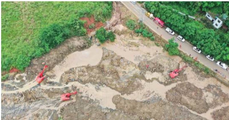
An aerial drone photo taken yesterday shows the rescue site of the flood-hit area after a heavy rainstorm hit Yongchuan District in Chongqing Municipality. – Xinhua
