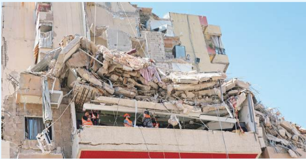
First responders yesterday inspect the rubble of a collapsed building following an Israeli airstrike a day earlier in Beirut's southern suburb of Haret Hreik. –AFP
