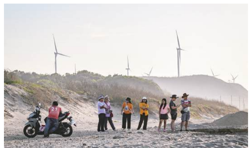
Wind turbines are pictured along the shore as seen from Bangui in the northern Philippines province of Ilocos Norte yesterday.
