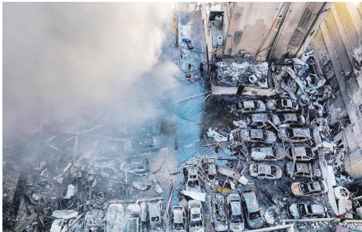
Firefighters attempt to extinguish a fire following an Israeli strike at the Corniche al-Mazraa neighbourhood of Beirut yesterday. – AFP
