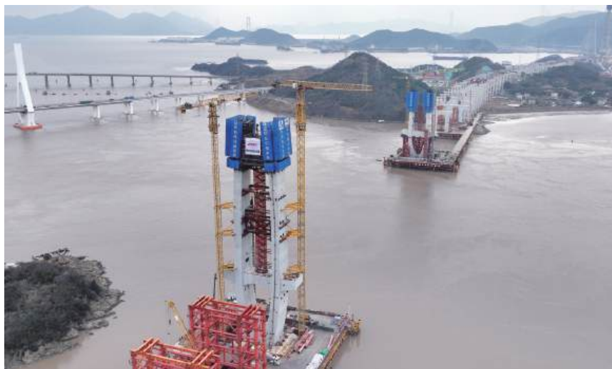
This aerial drone photo taken yesterday shows the concrete pouring site of the crossbeam on the east main tower of the Fuchimen road-rail bridge on the Ningbo-Zhoushan Railway in Zhoushan, Zhejiang Province. The concrete pouring operation for the crossbeam on the east main tower of the Fuchimen road-rail bridge was completed successfully yesterday, marking a breakthrough in the main tower's primary structure construction and laying a foundation for the subsequent construction of the entire bridge deck system. The Fuchimen road-rail bridge connects Zhoushan Island and Fuchi Island and is one of the key projects of the Ningbo-Zhoushan Railway. The bridge measures 1,726 meters in length with a main span of 388 meters, featuring a double-track railway and a six-lane expressway arranged on the same level. — Xinhua
