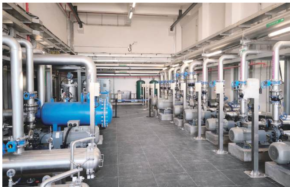
This photo taken during a media tour on Saturday last week shows pumping equipment in the newly completed first phase of the Coloane Reclaimed Water Station, located next to the Coloane Wastewater Treatment Plant. — Photo: Tony Wong
