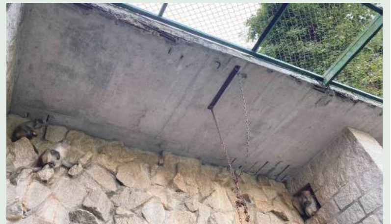
This undated handout photo provided by the Municipal Affairs Bureau (IAM) yesterday shows the concrete spalling and exposed steel beams in the macaque cages in Flora Park.
